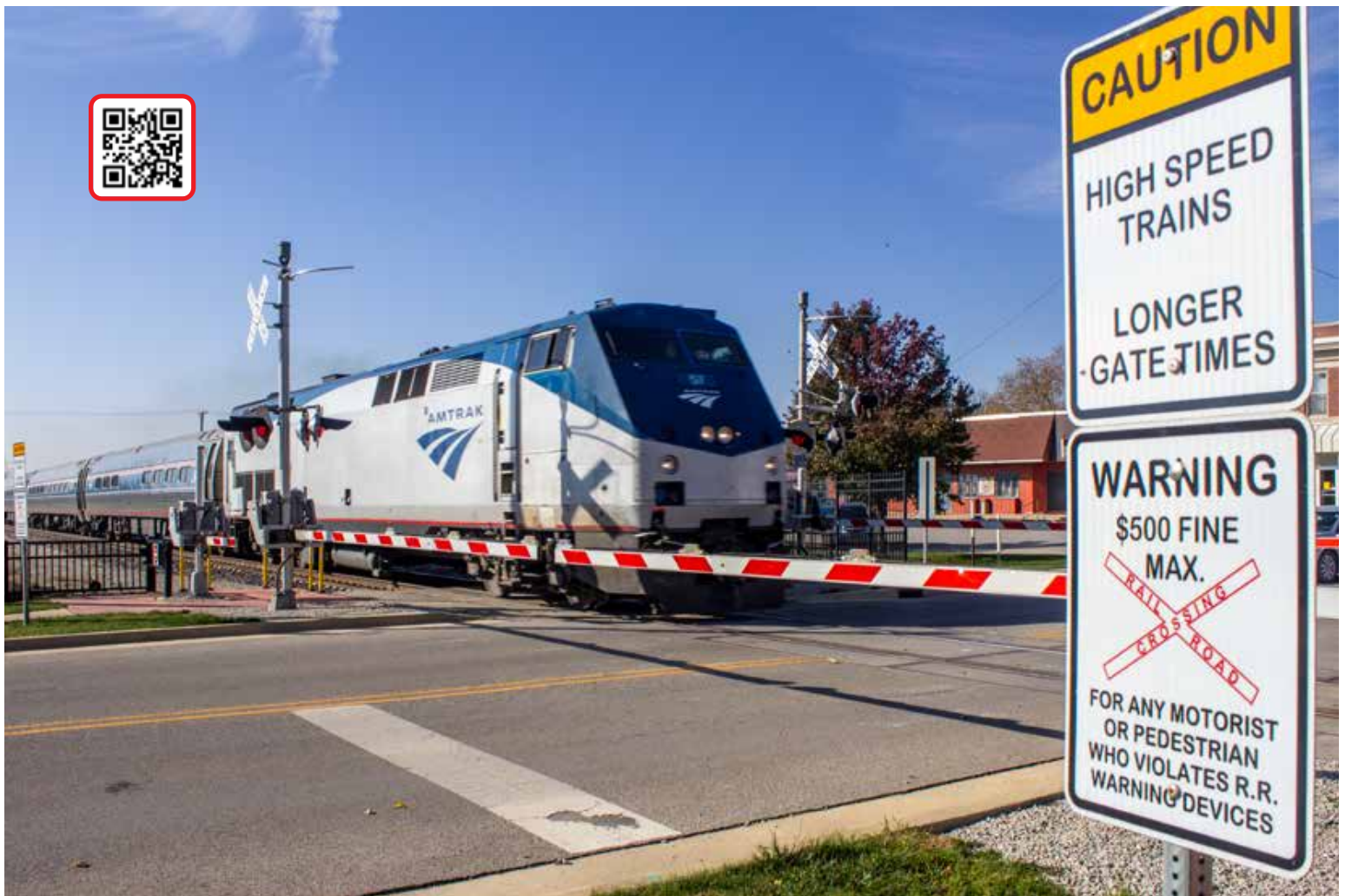
Four-quadrant gates, closed-corridor fencing, and additional signage warning of "longer gate times" protect a grade crossing in downtown Odell as Lincoln Service train No. 302 passes on Nov. 16, 2016. Two photos, Bob Johnston
